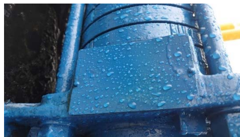
Fig. 2 Ex equipment installed in zone 2 but with its label plate being painted
